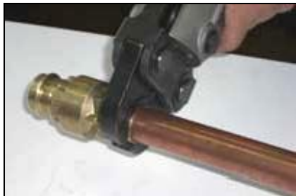
G. Open the jaw and place at right angles on the fitting. Visually check the insertion mark to ensure the tubing has not moved.
